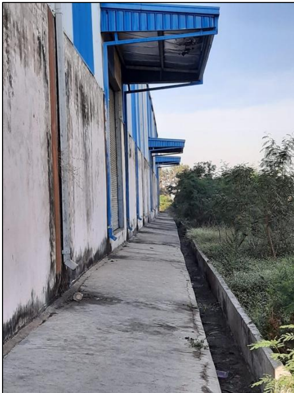
Rainwater channel Pipes installed at site
